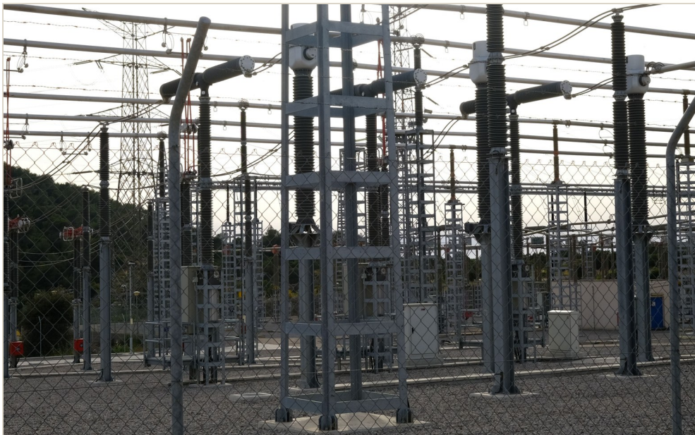
Grid connection is where projects stall. Interconnection and power systems specialists are the scarcest engineering profile in the region, and the shortage is sharpest in Singapore, Taiwan and South Korea.
