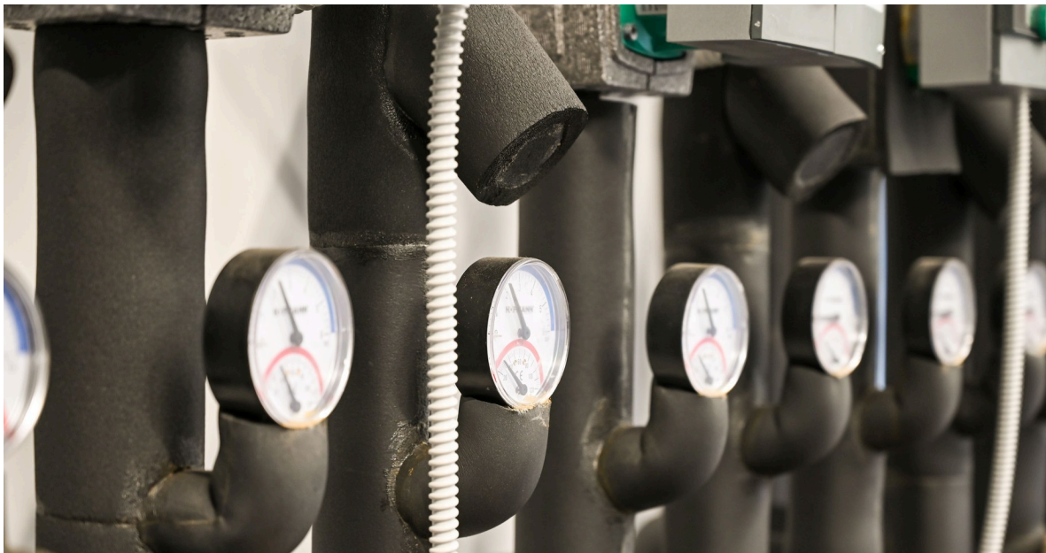
Insulated pipework and gauges. The paper argues that value is migrating towards the layers that outlast any one generation of compute.
